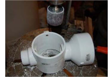
20. Sand pipes flush on the inside of the coupling.
